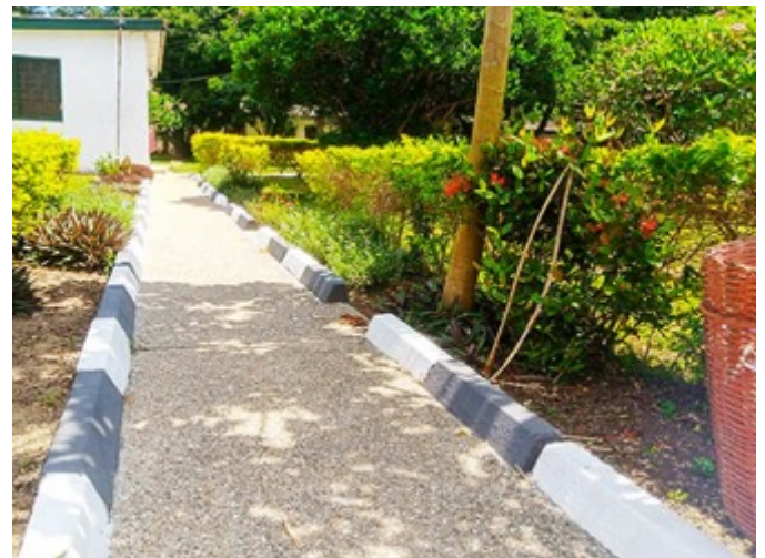
PPRC Campus – Painted Kerbs
