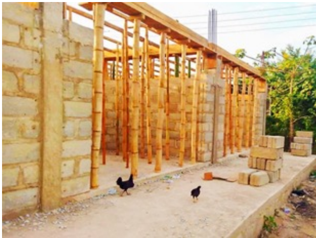
Shop Construction – making progress
