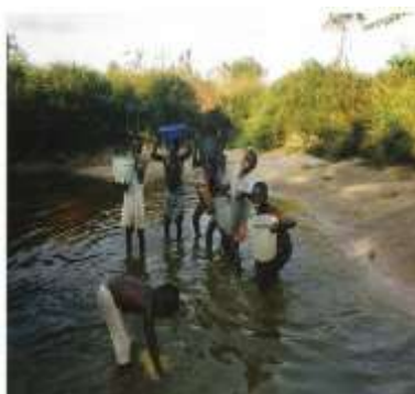
Children collecting water to add to the mortar mix
