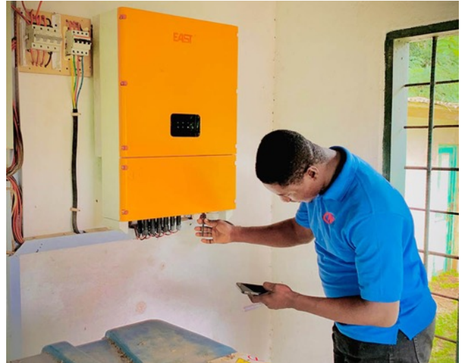
Solar Inverter – re-install
