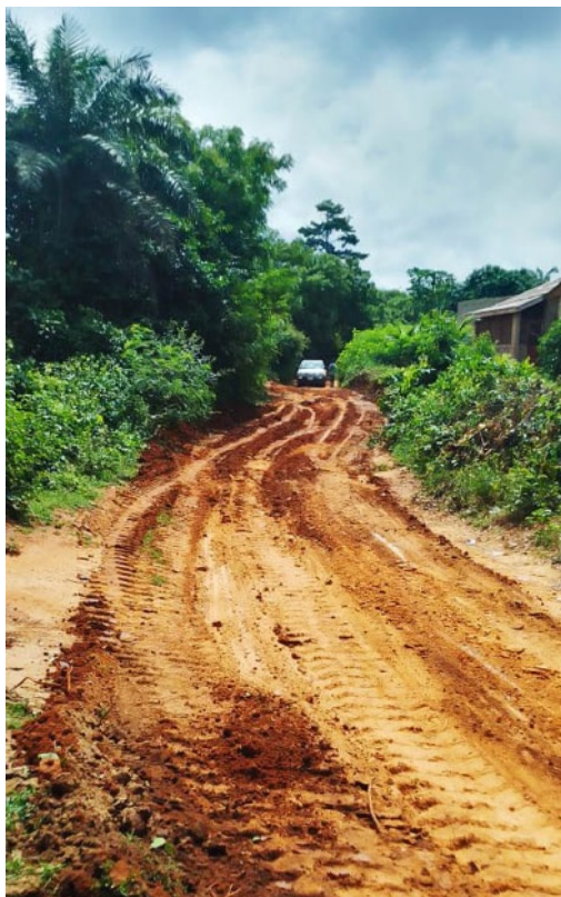
Local Roads – after repairs 1
