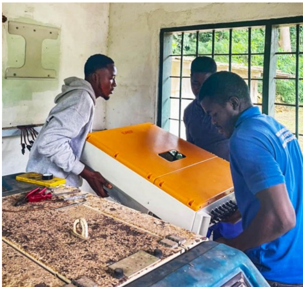
Solar Inverter – removal
